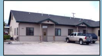
WWC's Helena, Montana office
