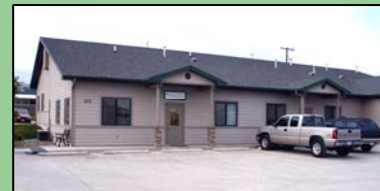
WWC's Helena, Montana office
