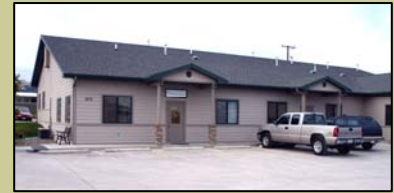
WWC's Helena, Montana office
