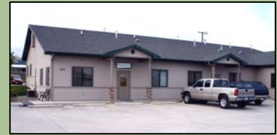
WWC's Helena, Montana office
